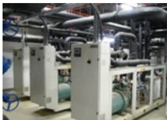
Geothermal heat pump at the Telenor House
