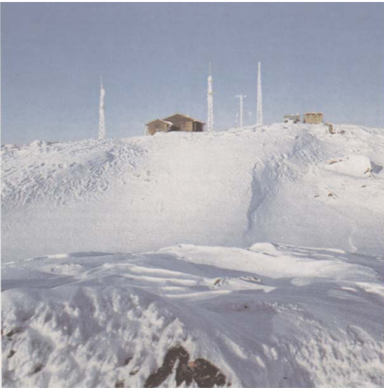
Radio link station for Oslo Lysverket in the Aurland mountains
