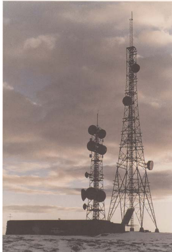
As a consequence of the major implementation of the digital radio link network, new masts had to be erected on several stations, as for instance at Ålfjell
