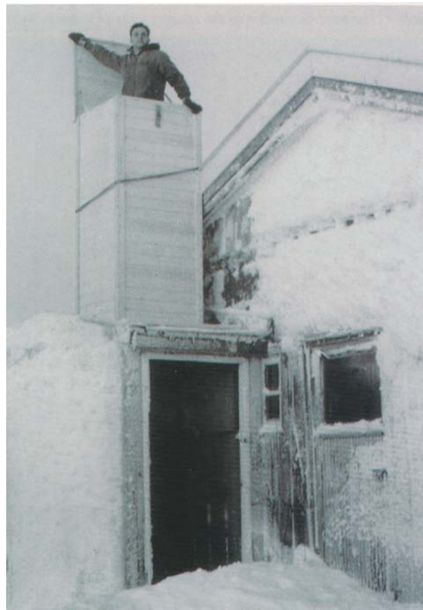
The snow was often 2 – 3 metres deep at the Kistefjell site in Troms 1004 metres above sea level. Therefore one had two entrances: One summer entrance through the door at ground level, and another winter entrance on top of the building
