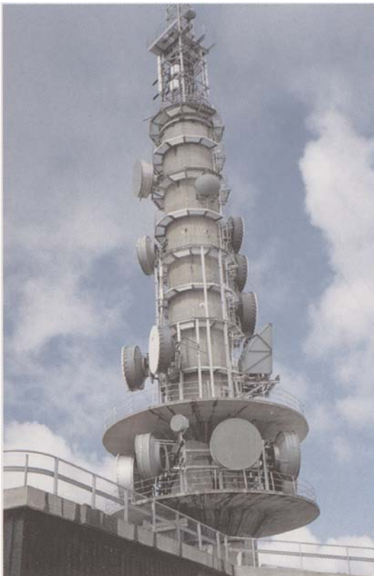
Antennas mounted on an antenna tower at Rønvikfjellet in Bodø 1988 (Photo: Truls Arnesen)
