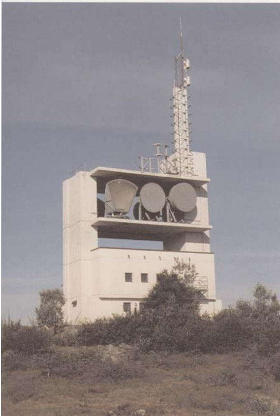
Tiffell radio link station in Trøndelag (From photo file of NØ.EA)
