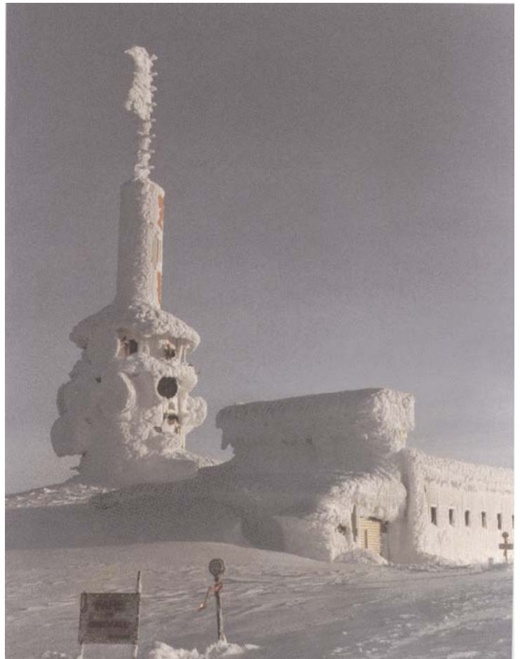
Storhogen radio link station at Sogndal 1173 metres above sea level, winter 1981 (From photo file of NØ.EA)
