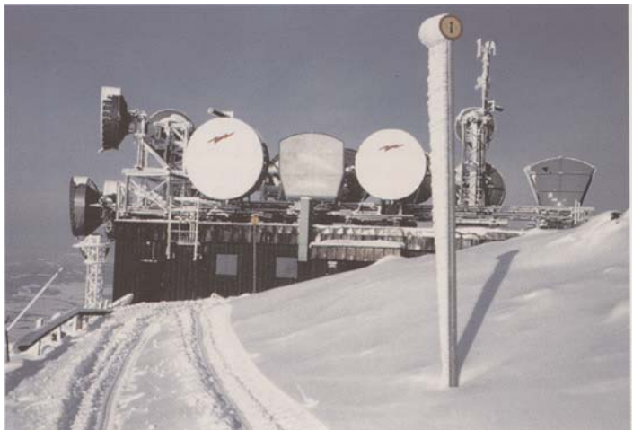
Vassfjellet radio link station in Trøndelag (Photo: Frank Aarhus)
