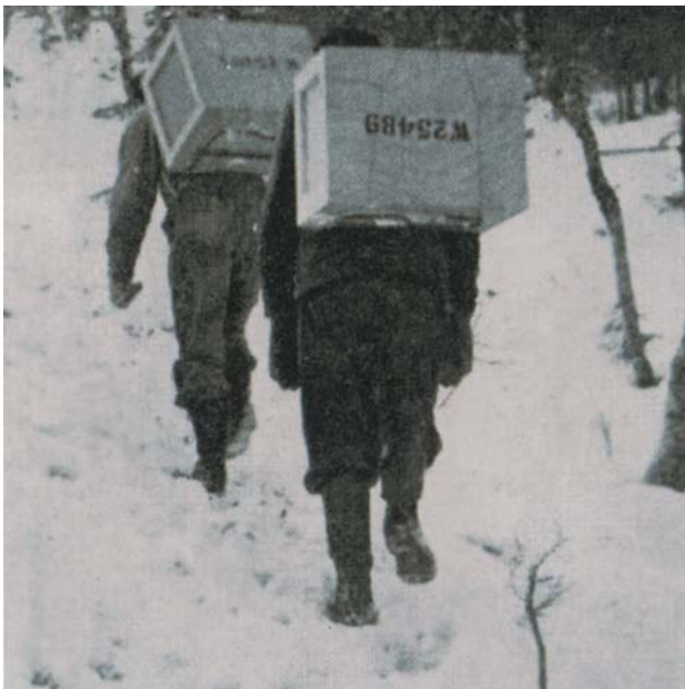
Power panels for the Marconi 48 channels VHF link are carried up to the site Offenåsen on the radio link between Steinkjer and Namsos in 1954
