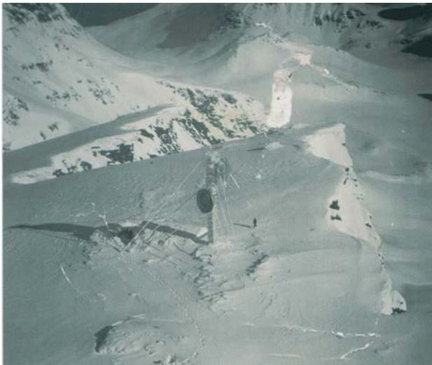
Hard to distinguish the details? Provisional site with 300 channels VHF link at Trolltind 924 metres above sea level on the Tromsø – Hammerfest link, 1963. The wind is pushed low by the mountain formation and a 2 – 3 metres deep heap of snow is formed
