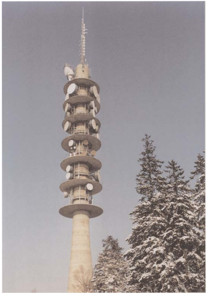
Røverkollen radio link station in Oslo, main station in the alternative radio link network (Photo: Frank Aarhus)
