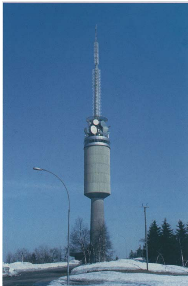
The Tryvann tower, Oslo, completed 1961
