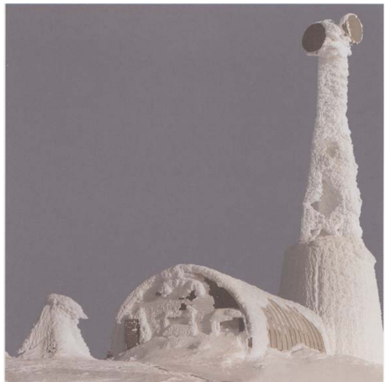
Andfjell radio link station at Saltfjell (From photo file of NØ.EA)
