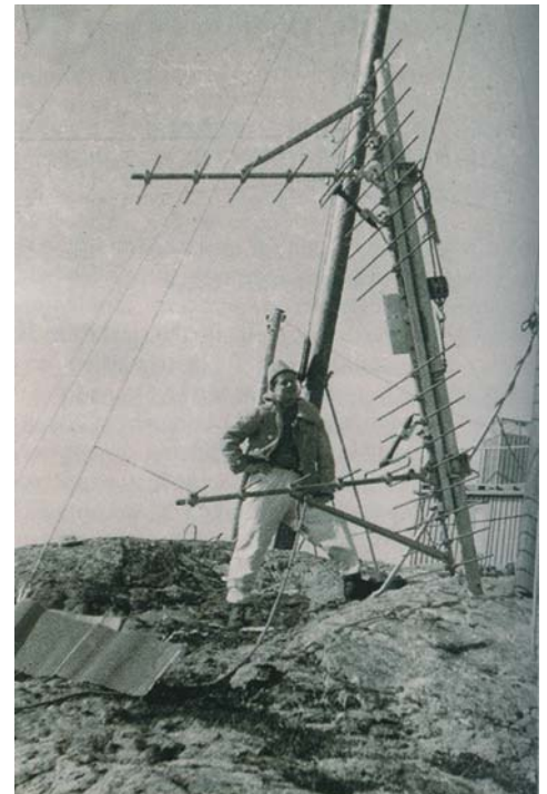
A VHF yagi antenna being mounted at the Falkhetta site near Rørvik on the Trondheim – Bodø link 1956
