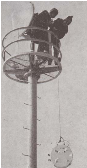
From the installation work in Drammen
