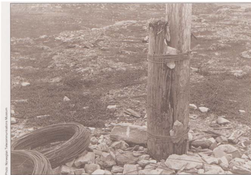
Broken telegraph pole – a picture of the ingenuity that had to be shown with the scarcity of resources in the reconstruction work after the Second World War, Finnmarksvidda in Northern Norway 1945
