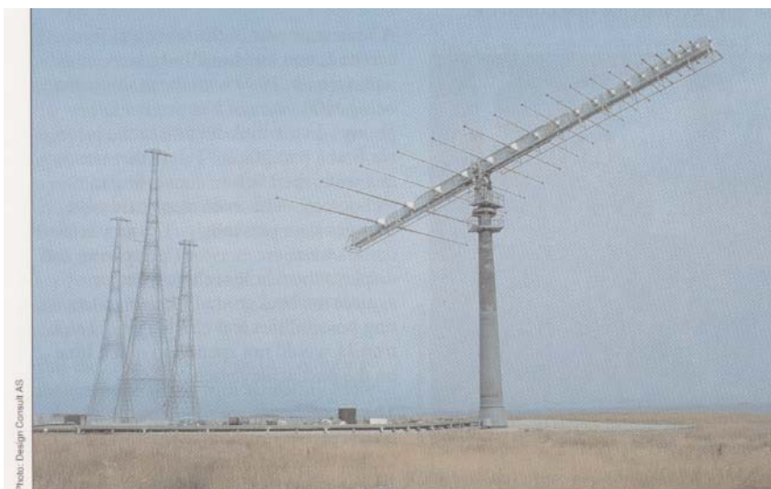
Medium and short wave antennas at Kvitsøy transmitting station, on the air from June 1982
