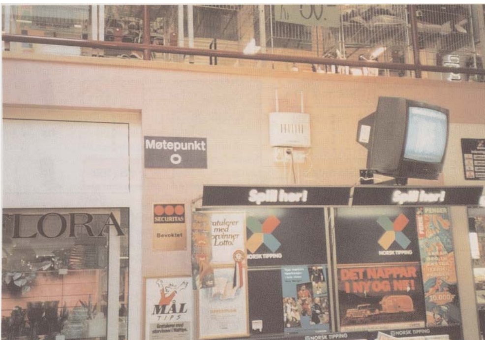
Figure 3 Base station site inside a shopping centre
