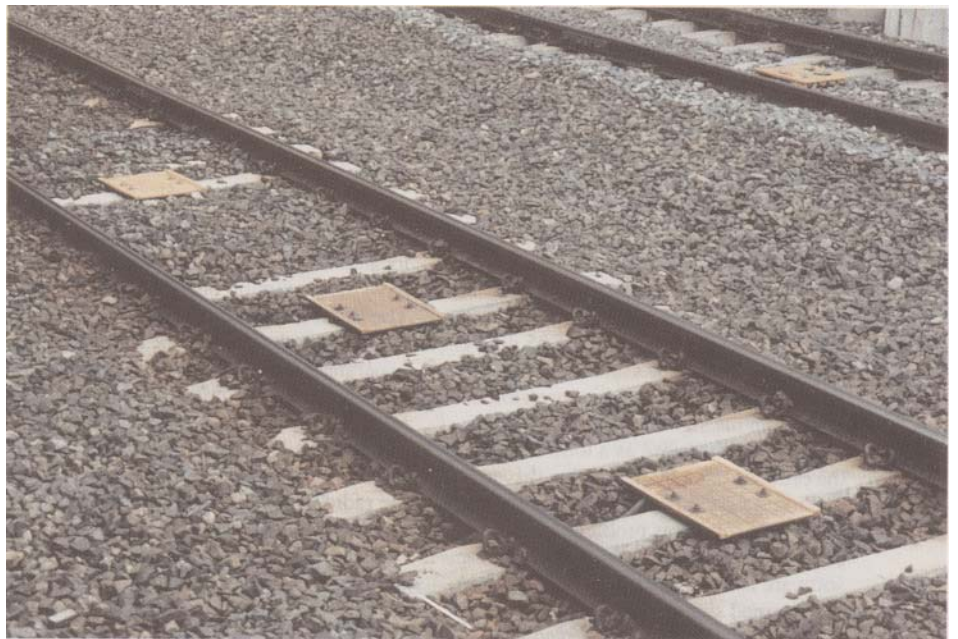
Figure 9 Balise (information points) located between the rails
