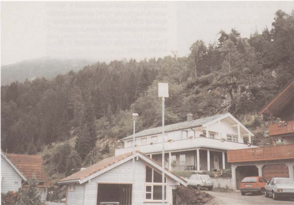
Figure 2 Typical base station installation in a residential environment
