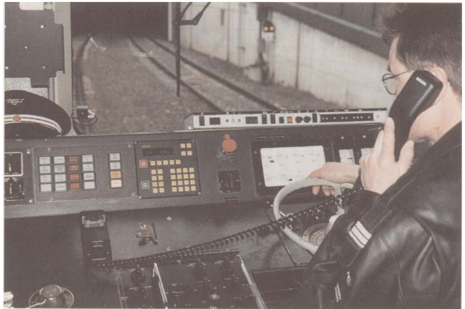
Figure 8 The Mobile Station control unit located in a train engine
