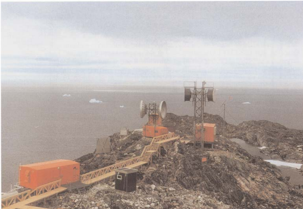
Figure 2 The new and the old repeater on NOKA
