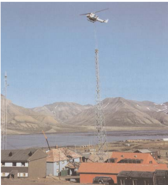
Figure 5 Top section of the new mast is put into place with the help of a helicopter
