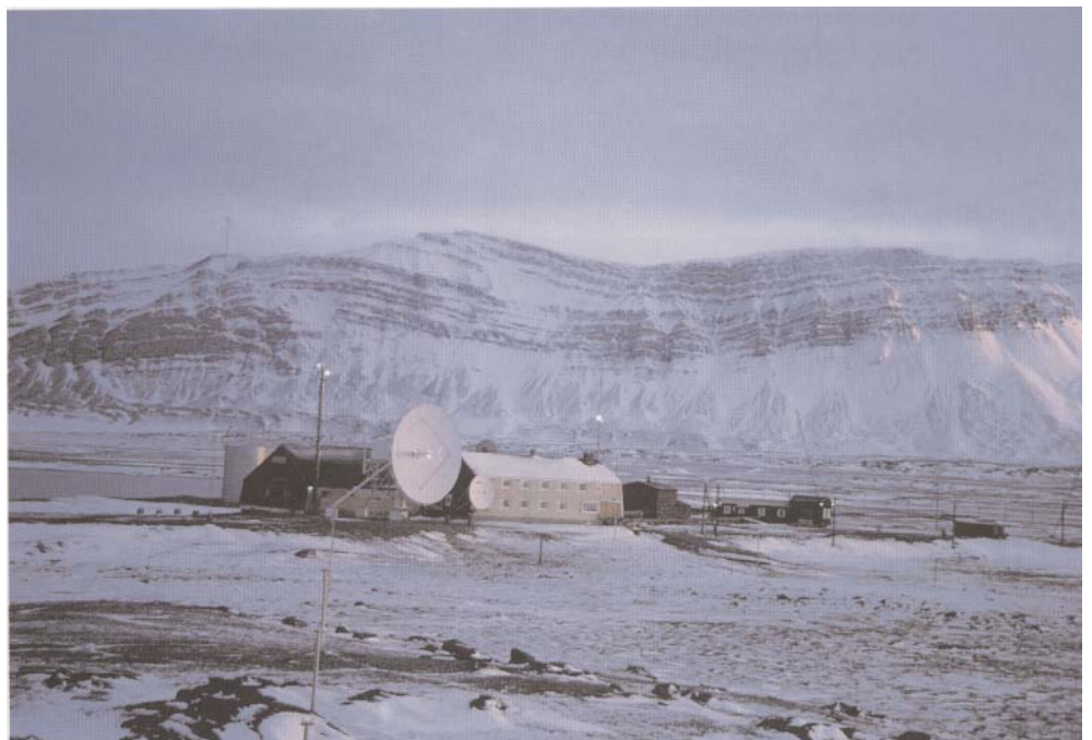
Figure 7 Isfjord Radio seen from the south-west. The earth station equipment is placed in the building on the left. The diesel tank can also be seen
