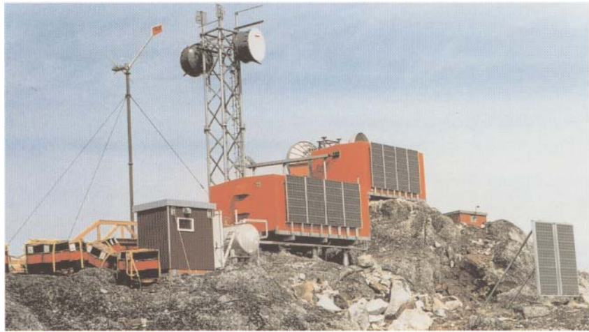
Figure 4 NUNA. The solar panels are mounted on the wall of the engine building facing south
