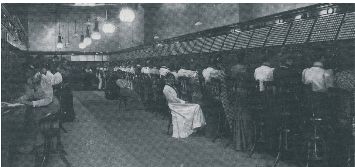
Manual telephone exchange (Bestorp, 1990)
