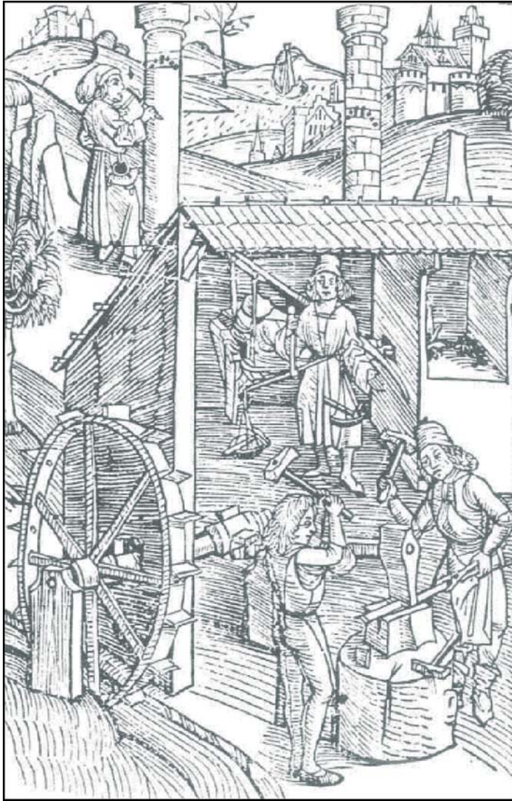
A water wheel from the 12th century. The illustration shows a trip hammer. Notice how the cams on the horizontal axis lift the hammer which then falls down heavily as the cams lose their grip due to turning (as used in Dahl, page 101, originally from Deutsches Museum in Munich)
