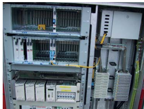
Figure 18 Access multiplexer installations in the Stavanger trial
