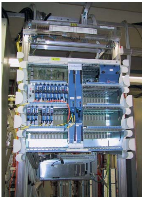
Figure 17 The broadband digital terminal installation in the Lura local exchange
