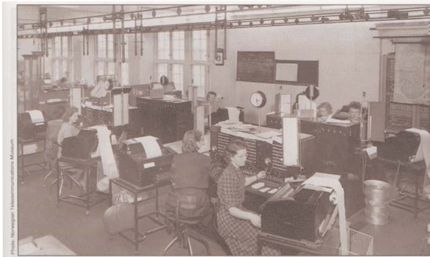
Manual telex exchange, Oslo 1952
