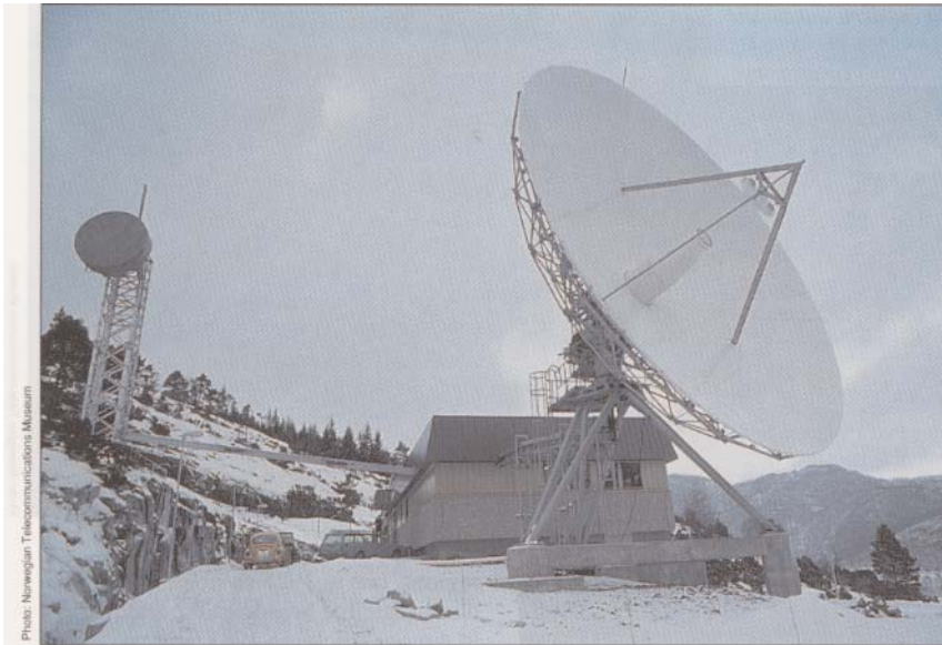
First in the world as a fully automatic INMARSAT coastal earth station, Eik in Rogaland was operational from 1982
